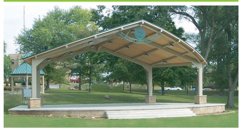
Poligon's Kokomo Amphitheaters (KMO) are four sided, amphitheater style shelters with a structural insulated panel (primary) roof for improved acoustics and a 4:12 pitch. \*Shown with optional ornamentation
